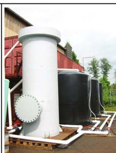
Figure 2. 25 m³/h sulfate-removal IX column.
