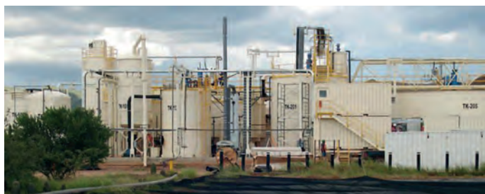
"SART comes in because it avoids the negative interference of base metals in the extraction of precious metals," BQE Water's David Kratochvil says
