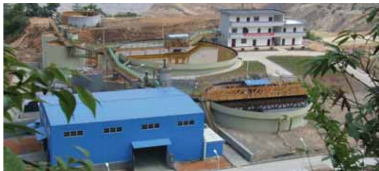
The Dexing copper mine where the ChemSulphide process is used to recover dissolved copper from mine water.
