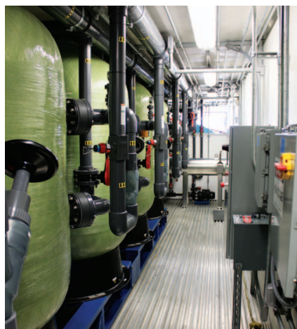
Met-IX™ plant produces treated water for discharge and a regenerant stream directed to a ChemSulphide® plant for nickel recovery.
