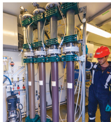
Mobile Selen-IX™ plant conducts field testing to remove selenium from wastewater.
