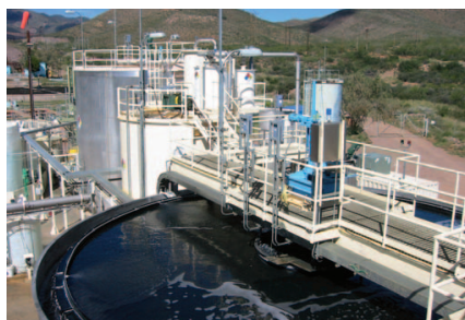
Sulphide precipitation plant that treats mine drainage and recovers dissolved copper.
