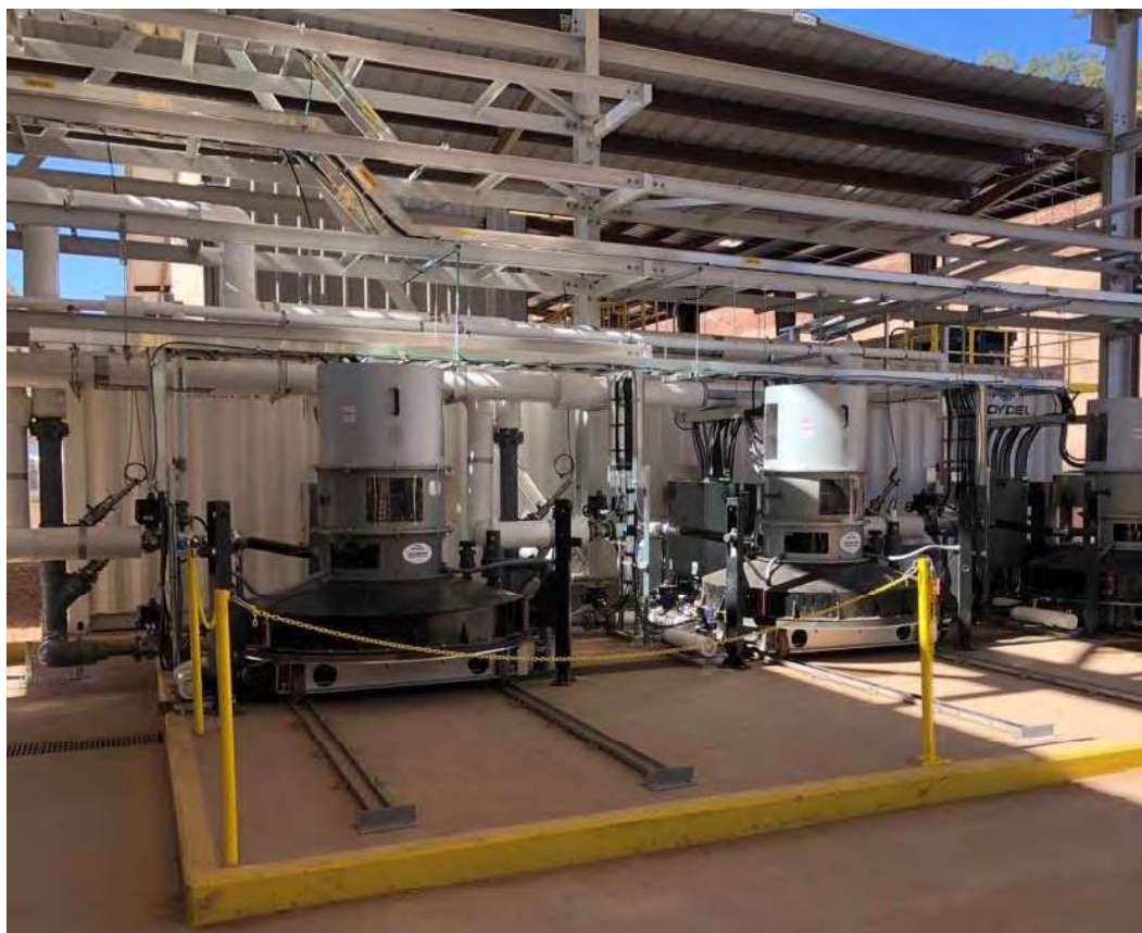
Figure 10: ERC with Constant-Gap Electro-Cells Applied to NF Retentate
